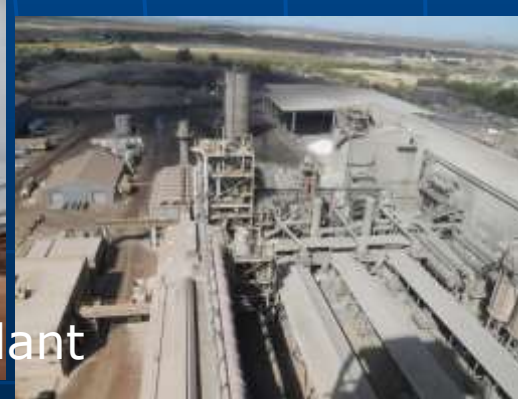
Rillito Cement plant
